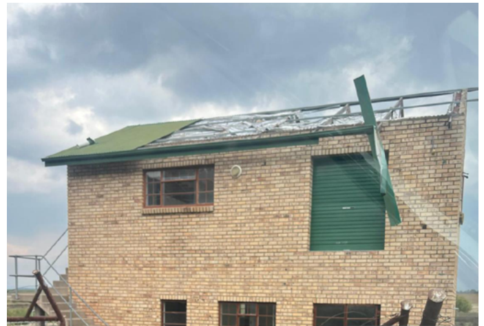
Ladybrand Waste Water Treatment Plant
